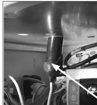
7. IMPORTANT! When re-mounting the new thermometer remember to properly seal the wire feed through.
