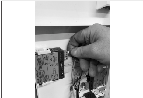
4. Pull gently the wire out from thermostat
