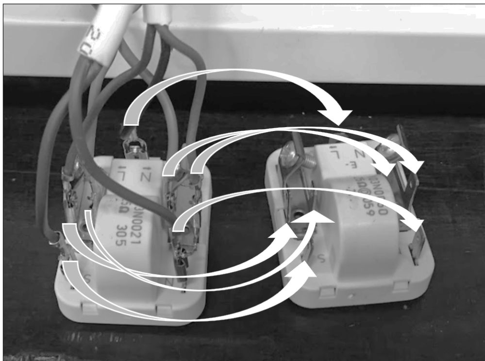
9. Exchange the wires 1/1 from the old starting device to the new one.
