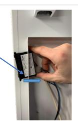
10: Use your finger to press/slide the back the fixing clamps to fasten the thermostat body
