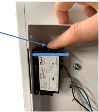
5: Use your finger to press and slide the lower clamp backwards to remove from the thermostat body
