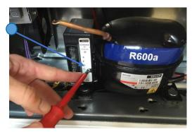
4: Place a screwdriver in the small vent in the plastic cover
