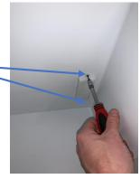
2: Unclip the sensor probe from the fixation clamps
