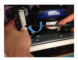
6: Use a screwdriver to disconnect the socket from compressor
