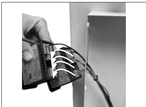
7. Switch the wires from old to new thermostat one by one
