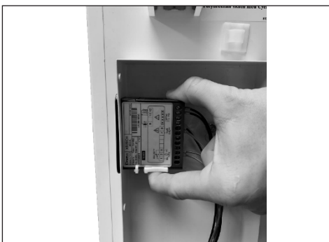
10. Use your finger to press/slide the back the fixing clamps to fasten the thermostat body
