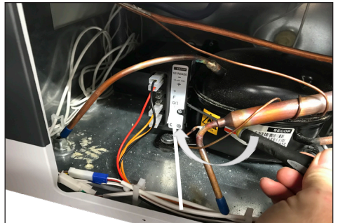
4. Unclick plastic cover/starting device from compressor bracket
