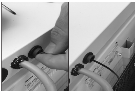
5. Push the antenna wire through the wire entry
