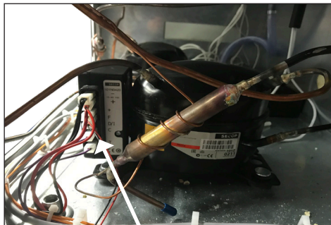
1. Dismount the 6 wires from ECU. Grab the wire socket and pull gently.
