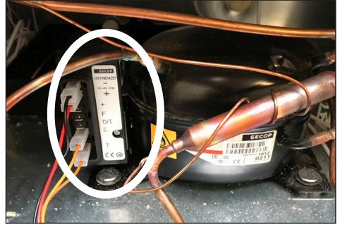
The starting device is mounted to the left side of the compressor.
