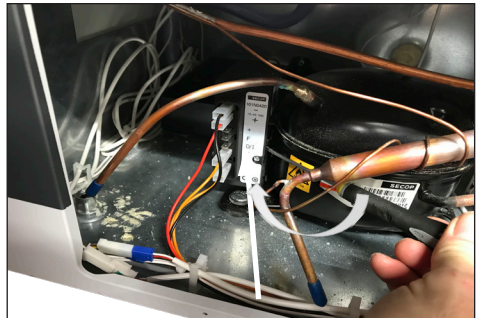
4. Unclick plastic cover/starting device from compressor bracket
