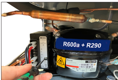
2. Loosen the screw a couple of turns.
